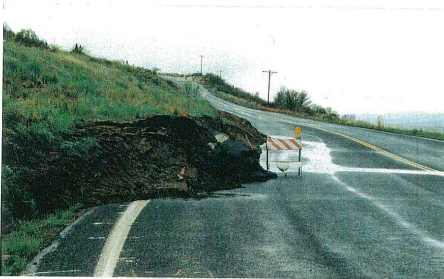
Photo 3. Toe of landslide encroaching on Mesa Road. Note white stripe on asphalt chunk in toe bulge left of barricade.
