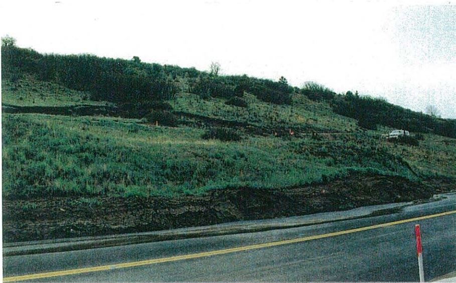
Photo 1. Landslide above Mesa Road near 30th Street. Note van (upper right) parked on bike path. Scarp in upper middle part of photo. Toe encroaching on Mesa Road.
