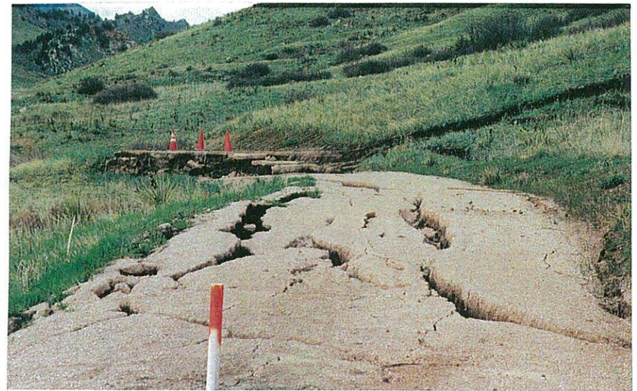
Photo 2. Bike path, damaged and offset by landslide, above Mesa Road. Note traffic cones in the background, on top of in-place path.
