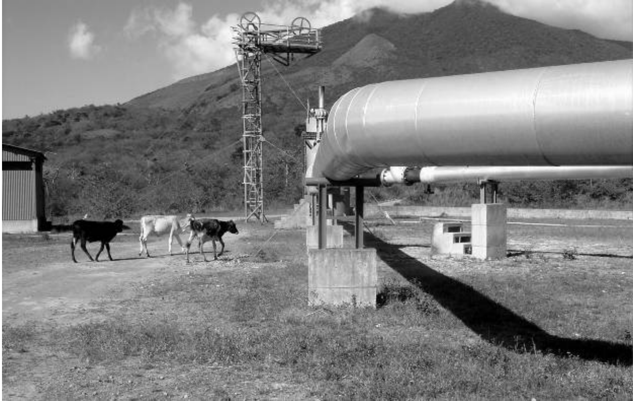
Typical Geothermal Pipelines, at the Miravalles Geothermal Power Plant, Costa Rica. These pipelines are elevated to allow cattle free access to pasture. 17
