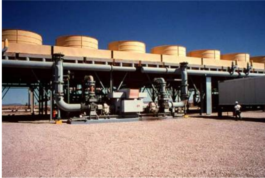
Soda Lake II Power Plant, Nevada. Two binary-cycle air-cooled units producing a total of 12 MW. The two units are seen in the foreground; the air cooling fans are at the top (yellow); a geothermal pipeline is visible in the background to the left. 18
