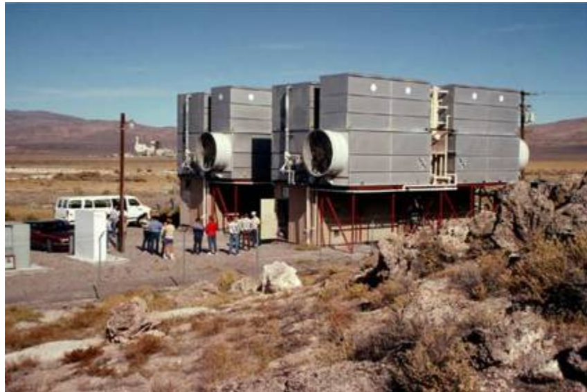
Binary Power Plant at Wendell-Amadee, California. This unit produces 1.9 MW and is air-cooled: the air-cooling units are the large grey structures in the top of the plant. This plant runs automatically and calls an operator to come to the site if a problem is detected. 18
