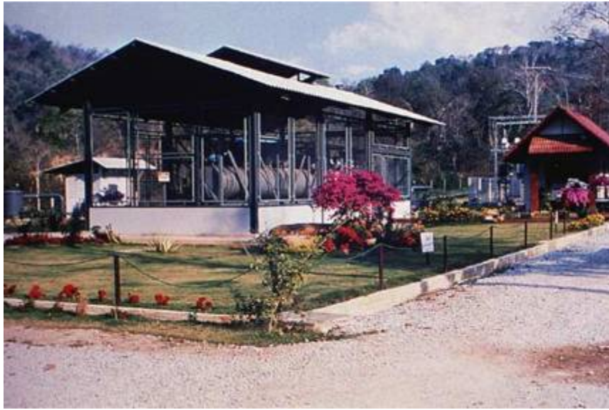
300 kW Binary Power Plant at Fang, Thailand. After passing through the heat exchanger in the binary power plant, the geothermal water is cascaded for use at a refrigeration (cold storage) plant, for crop drying, and at a spa. 18,19
