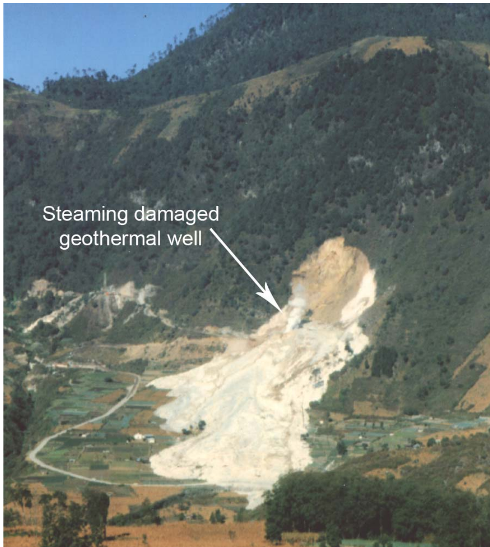
Landslide at Zuni Geothermal Field, Guatemala, probably at least partially caused by poorly designed geothermal extraction well field. 24
