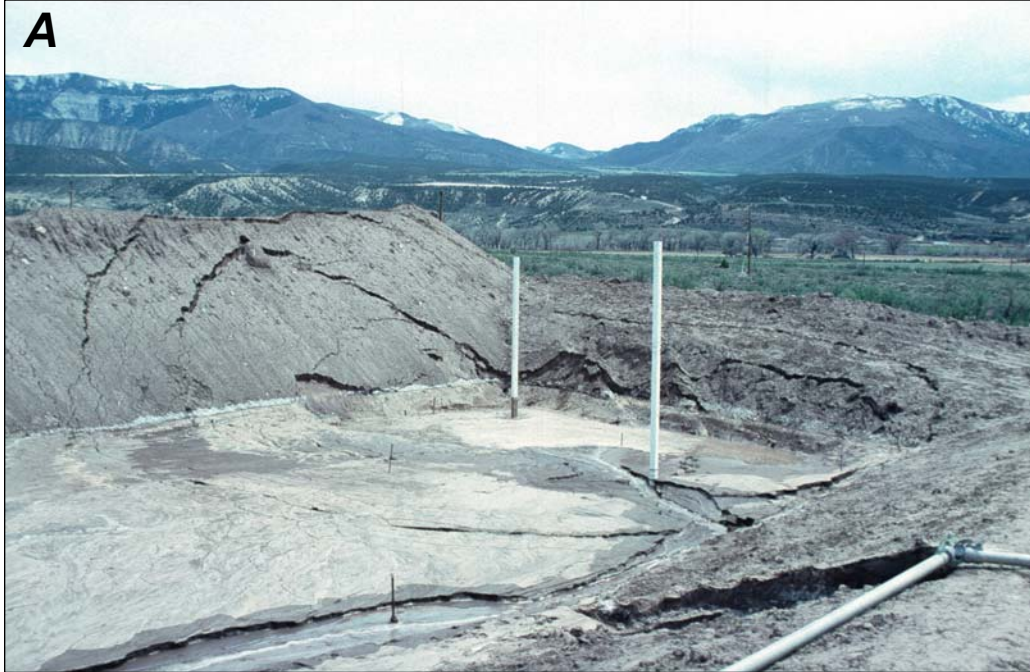
Figure 4-4. Ground settlement at test ponds along the proposed Interstate 70 alignment west of Rifle during preliminary studies in the mid-1970s. Site is on a large alluvial fan on the north valley side of the Colorado River. Note arcuate cracks and subsidence of test embankment. During the test, the ponded water sometimes completely drained into a network of pipes formed in the subsurface soil. Photos courtesy of R. Barrett and CDOT.
