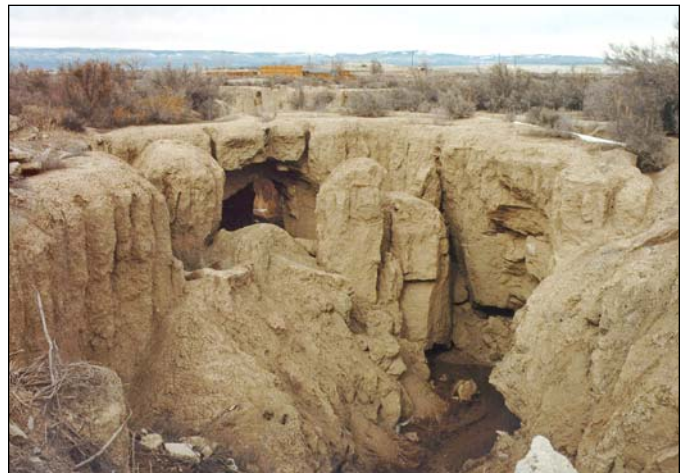
Figure 5-13. Soil dispersion and piping voids may create soil bridges. North of Montrose, progressive collapses of a large piping void, which had become essentially a subterranean drainageway, has created a tributary of Loutsenhizer Arroyo that is spanned by the soil bridge, which is about 8 ft long.
