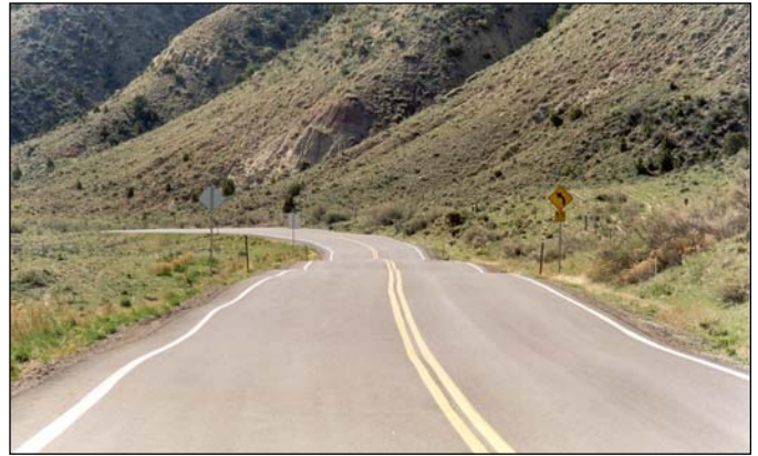
Figure 7-17. Settlement distress on State Highway 64, between Meeker and Rangely, where it crosses over coalesced, collapse-prone alluvial-fan and hillside colluvial soils on the floor of the White River valley.
