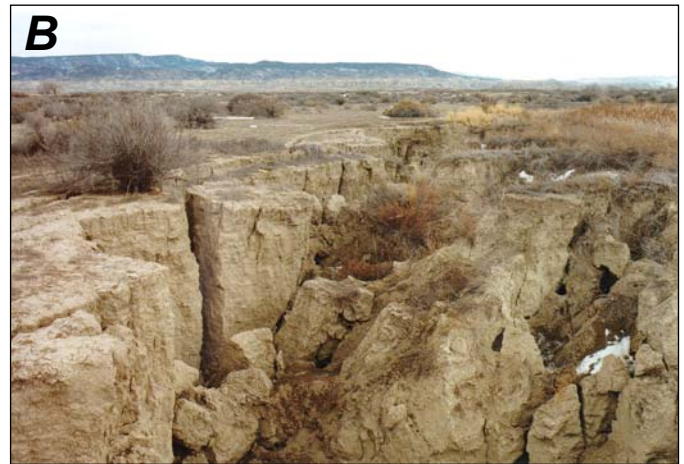
Figure 5-12. Erosion damage caused by piping that may occur from uncontrolled flows of water. This pseudokarst terrain was the result of irrigation runoff from an adjacent field near Loutsenhizer Arroyo, north of Montrose.
