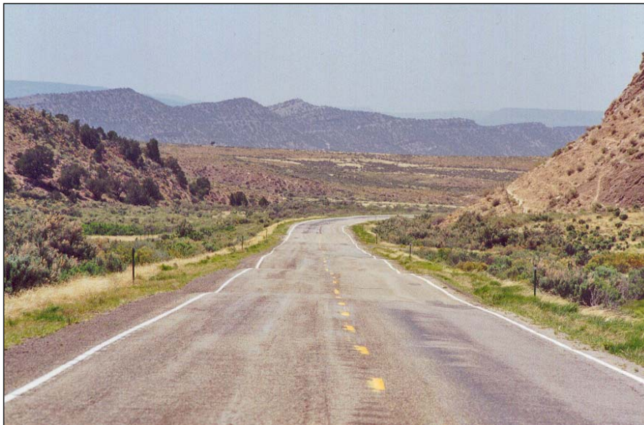
Figure 7-11. State Highway 141 shows settlement distress related to hydrocompaction where it enters Big Gypsum Valley and passes over collapse-susceptible alluvial fans and Big Gypsum Creek alluvium (low-relief, vegetated areas on the left and right of the road). Evaporite (gypsum) bedrock is exposed on the hill to the right.
