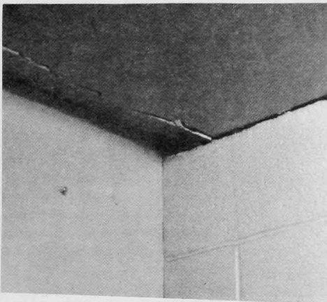
Figure 7. Cracked ceiling in Boulder school district building caused by 2 in. of uplift on left wall.
