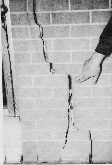
Figure 6. Cracked brick wall at Ridge Home caused by swelling clay.
