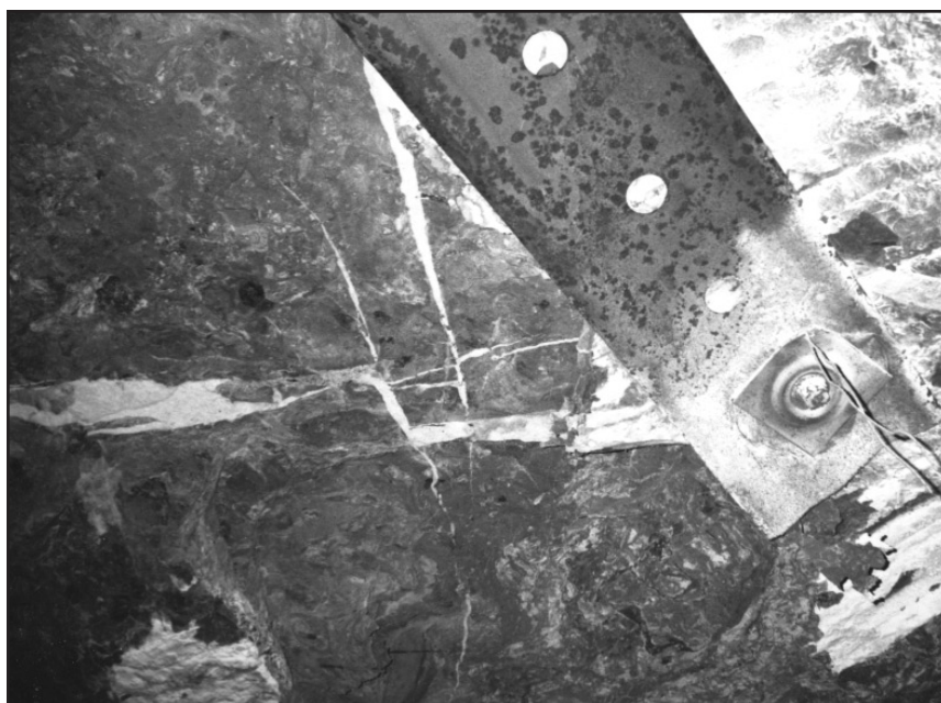
Figure 16. Photograph showing a cross-hatch pattern composed of small, intersecting dikes in the roof of the Cameo Mine and that resemble infilled fractures.
