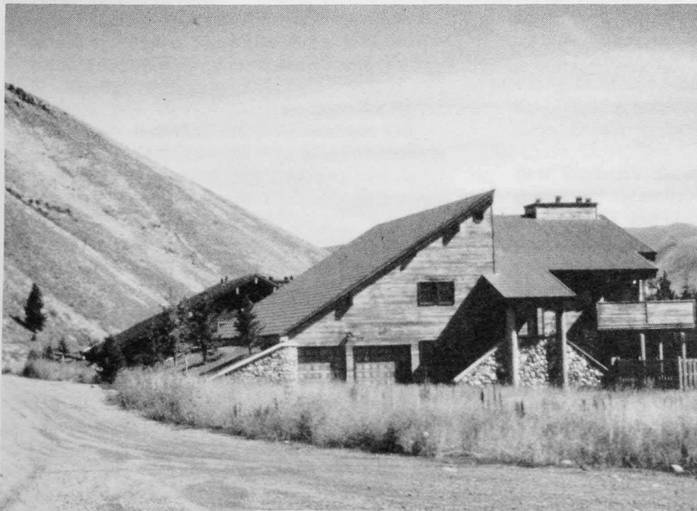
*Figure 33. This ramp roof in Ketchum, Idaho faces toward the avalanche direction. The small deflection angle reduces avalanche dynamic loads.*
