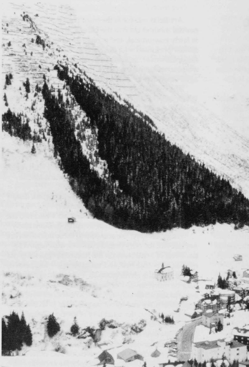
*Figure 27. Supporting structures are built across the avalanche starting zone above this Swiss village. The structures are nearly continuous across the slope to prevent small avalanches from flowing between structures.*
