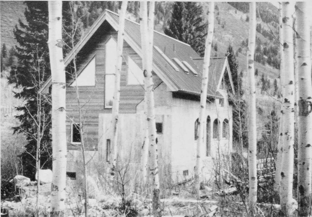
*Figure 34. The reinforced uphill corner of this house near Aspen, Colorado is oriented toward the avalanche direction and acts as a splitting wedge.*
