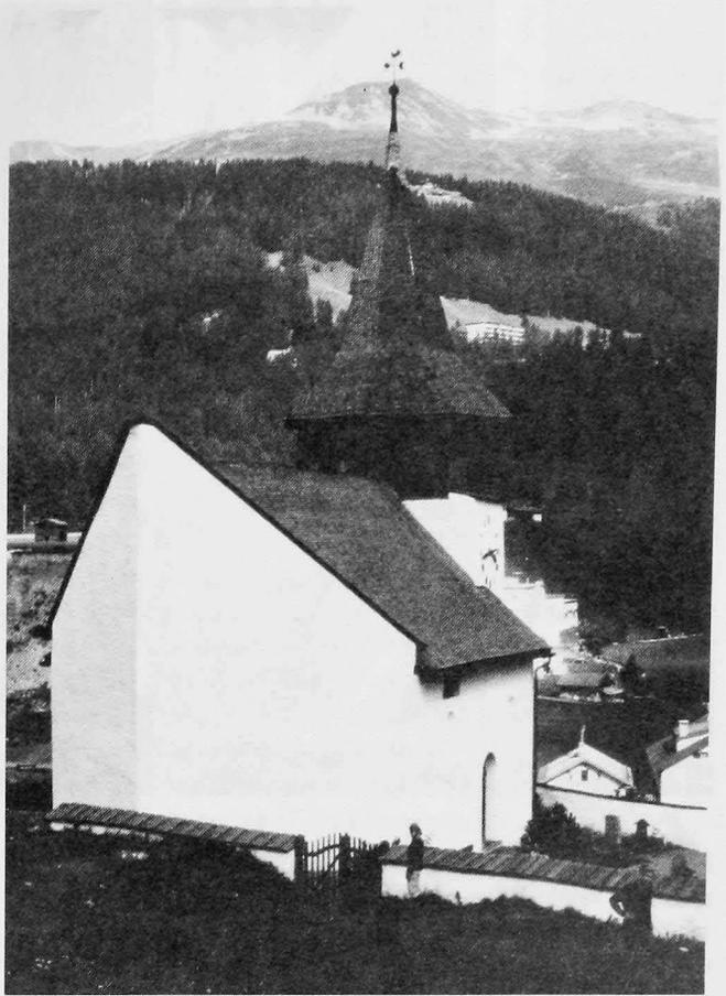
*Figure 32. The splitting wedge on this Swiss church deflects avalanches laterally, reducing normal forces.*
