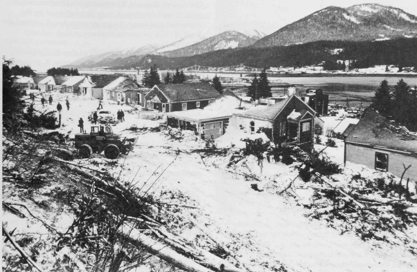
*Figure 11. The extensive damage to this subdivision in Juneau, Alaska, was caused by a dry-snow/powder avalanche. The energy of the fast-moving, low-density flow and entrained debris produced the damage. Thick, dense deposits of avalanche debris did not overrun the site.*
