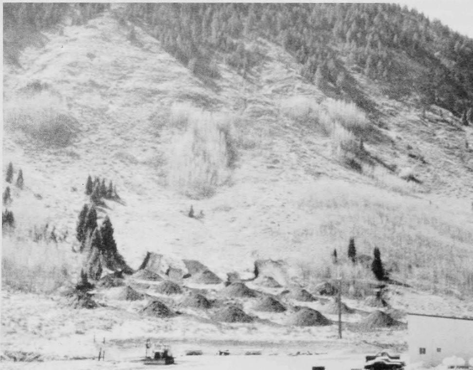
*Figure 31. The uppermost row of mounds are located on a slope of  $15^\circ$ , where avalanche begin to decelerate naturally. Four rows of mounds have been used in this case to provide protection from the "10-year" avalanche.*
