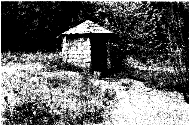
Figure 111.--Trimble Hot Springs. Spring is inside rock house.
