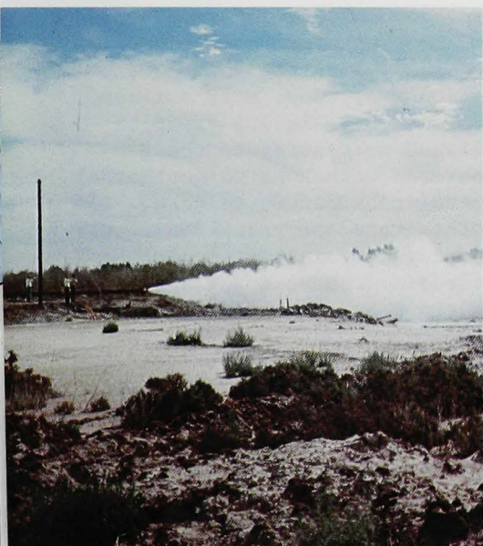
Figure 4. Testing a recently drilled geothermal well at Cerro Prieto, Mexico.
