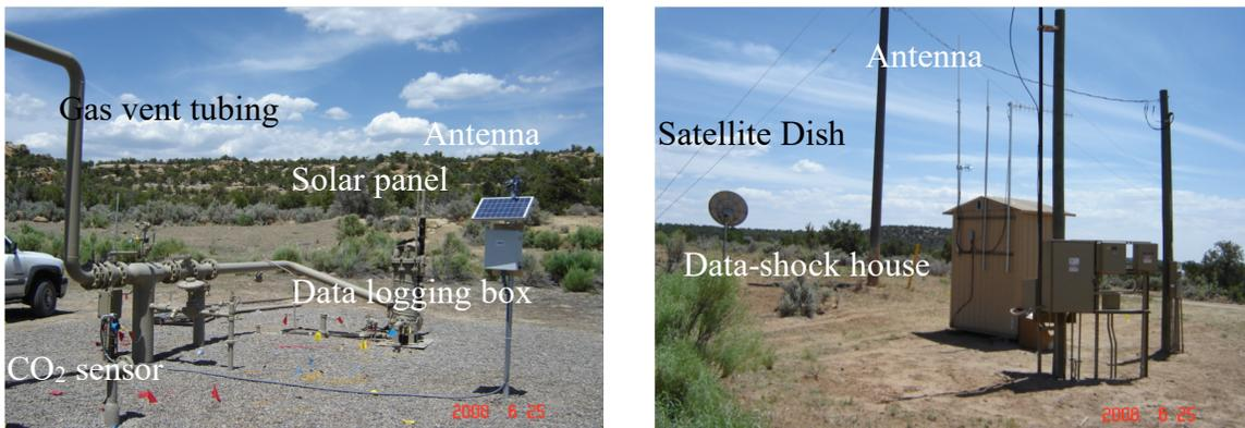
**Figure 11: The CO<sub>2</sub> Sensor Installed at the FC STATE COM Well**
