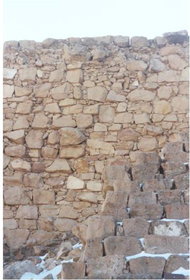
Figure 13. Exposed downstream face of upstream masonry wall. A small portion of downstream shell is evident in lower right of photo
