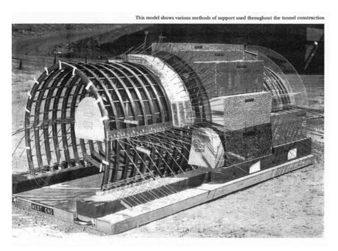
Figure 8. Conceptual model of tunneling method for I-70 bores through the Continental Divide.
