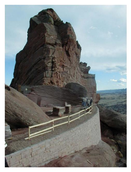
Figure 13. The MSE wall follows the natural topography in an arc facing Mt. Morrison to the west.
