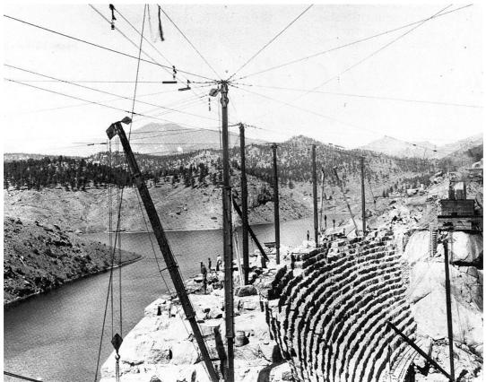
Figure 4. View of Aerial Tramways During Construction of Cheesman Dam.
