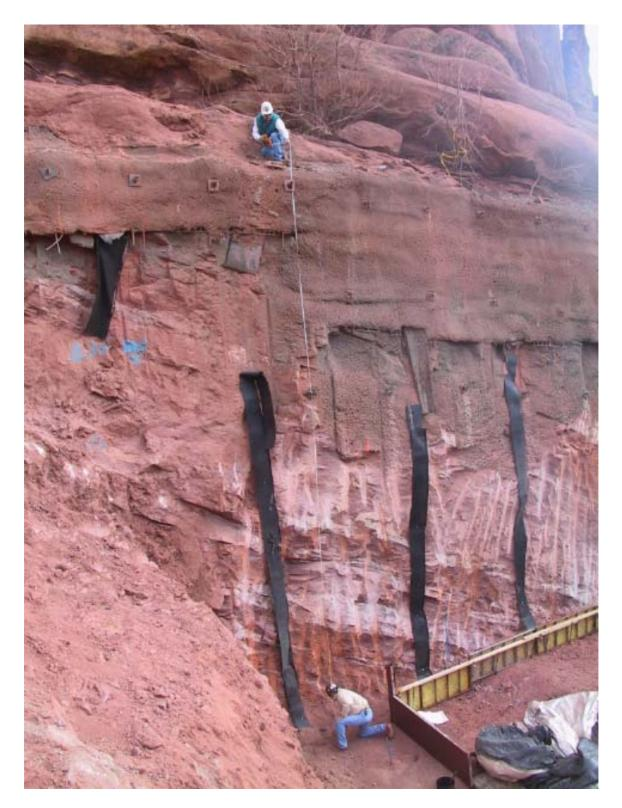
Figure 11. Soil nails were used to stabilize the 35-ft high cut during construction of the new Visitor Center at the top of the amphitheatre.
