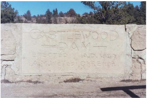
Figure 19. Large rhyolite dedication block. Note contrast between edges of rhyolite and adjoining conglomerate blocks.
