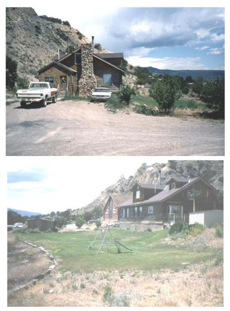
Figure 16. The front (lawn side) of this cabin is settling, apparently due to collapse of soils and dissolution of gypsum from irrigation of the lawn.
