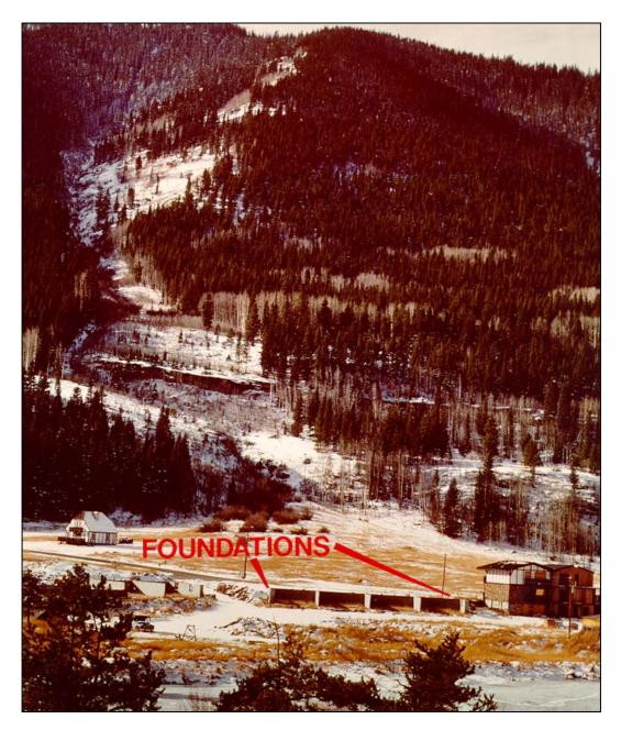
Figure 16. An avalanche path in Vail, Colorado. A forested initiation zone and a well-developed central chute and runout zone are visible. Houses within the runout-zone fringe have been built with reinforcement for design-avalanche loads. Photo from Colorado Geological Survey.
