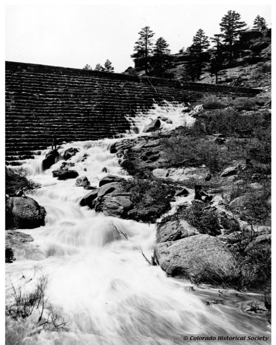
Figure 7. High amount of seepage through dam on left abutment, prior to reconstruction. Outlet pipe is just out of view to left of photo (Colorado Historical Society).
