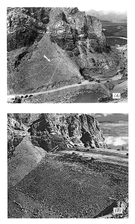
Figure 2. Views before (A) and after (B) construction of Taylor Park Dam, central Colorado. Note talus deposit that serves as the right abutment of the dam, and the chalk line (white arrow) at the left center of photograph (A) showing the location of the right end of the future dam on the talus cone. (1937 photographs by A.A. Whitmore, U.S. Bureau of Reclamation)
