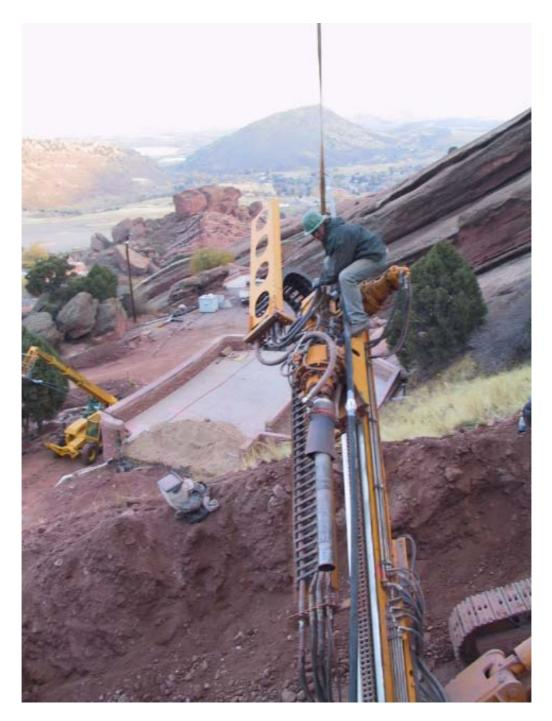
Figure 18. Ground anchors were installed to stabilize the south slope and keep the planters along the amphitheatre seating shored during construction.
