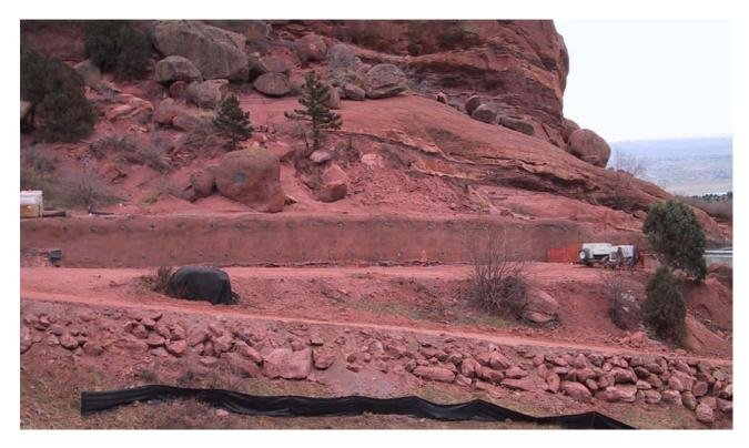
Figure 9. The concourse ramp cut was stabilized using soil nails.
