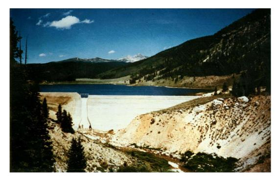
Figure 5. Downstream view of the completed project. Note the raised crest sections at either end, the pre-existing service spillway, the extended outlet conduit (in operation), and the RCC auxiliary spillway liner.
