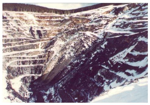
Figure 4. Northeast corner slope failure — March 1983.
