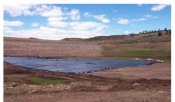
Figure 16. In October of 2002, an upstream blanket was placed along the reservoir bottom just south of Horsetooth Dam (U.S. Bureau Reclamation photo).
