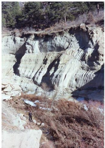
Figure 2. Right abutment slopes downstream of dam, showing excessive erosion in Dawson Arkose during and following failure. Note near vertical slopes in sandstone and less steep slopes in center mudstone
