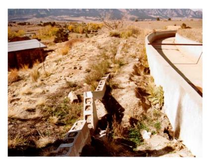
Figure 4. Compression associated with subsidence has upended the cinder block wall. Marshall area, Boulder County.
