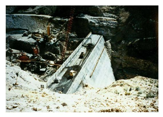
Figure 8. RCC placement in the upper part of the dam as viewed from downstream high on the right abutment. The work area with batch plants, conveyors, and crane can be seen at the left. The complete RCC placement sequence of delivery, spreading, and compaction can be viewed. Note the stepped downstream facing and safety barriers.
