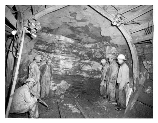
Figure 2. Lemon Dam - Red siltstone of the Cutler Formation exposed in the outlet works tunnel.
