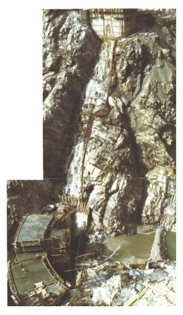
Figure 2. Excavation for Keyway on Left Abutment.
