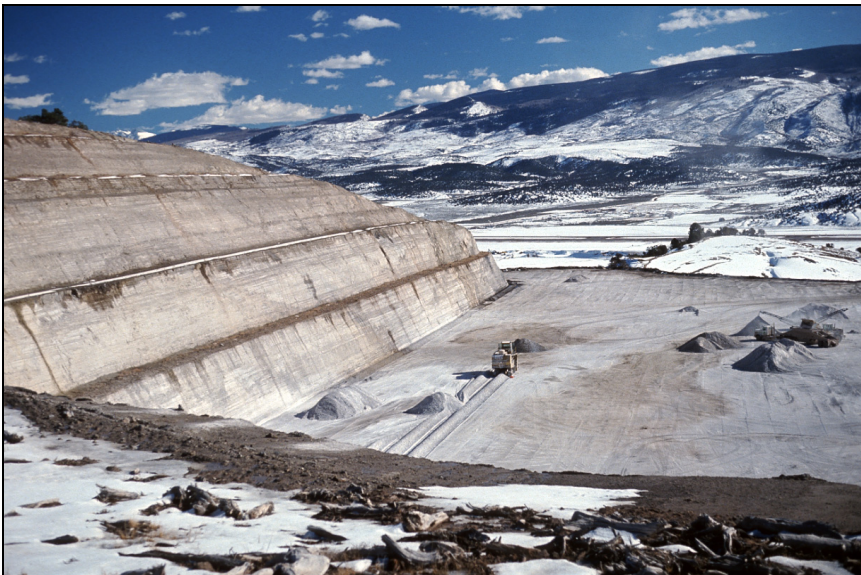
Figure 14. American Gypsum Quarry, Gypsum, Colorado. Pavement profiler is cutting furrows in the center of the photo. (Photo by John Keller)
