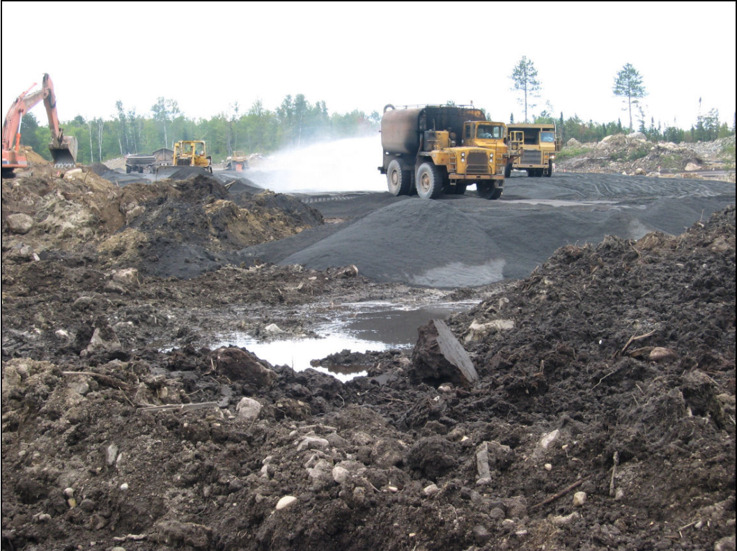
Figure 20. Coarse taconite tailings used as granular fill, U.S. Highway 53/169 interchange project (photo courtesy Kurt Johnson, NRRI).
