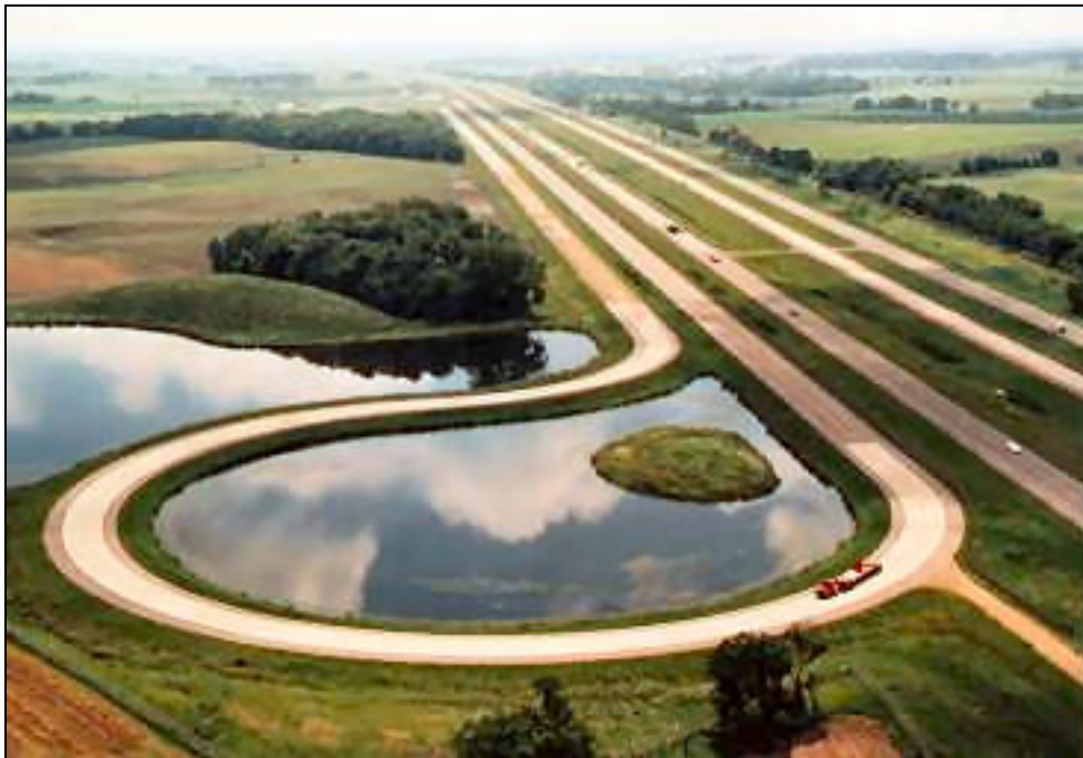
Figure 16. Mn/DOT's MnROAD test facility in Albertville, MN, showing low-volume test road in foreground (loop) and I-94 to the right (photo source: Mn/DOT).
