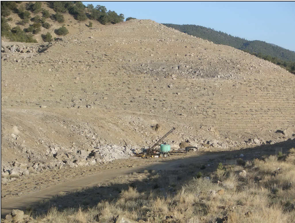
Figure 11. Looking west at five-year-old contour furrows constructed through bedrock outcrop zone of slope. April photo only shows shrub development.
