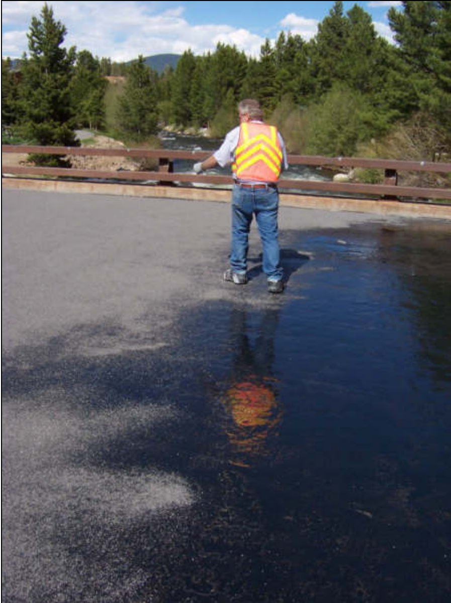
Figure 18. Fine taconite aggregate being applied as a friction coarse to a Frisco, CO, bridge deck in May, 2006 (photo source: Superior Coating Specialists, Proctor, MN).
