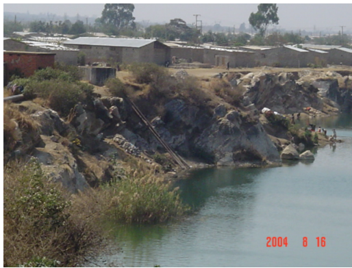
Figure 11. A dolomitic marble quarry filled with water and near an unplanned settlement in Lusaka. This quarry was operated by a large company (Crushed Stone Sales Ltd) before being abandoned.
