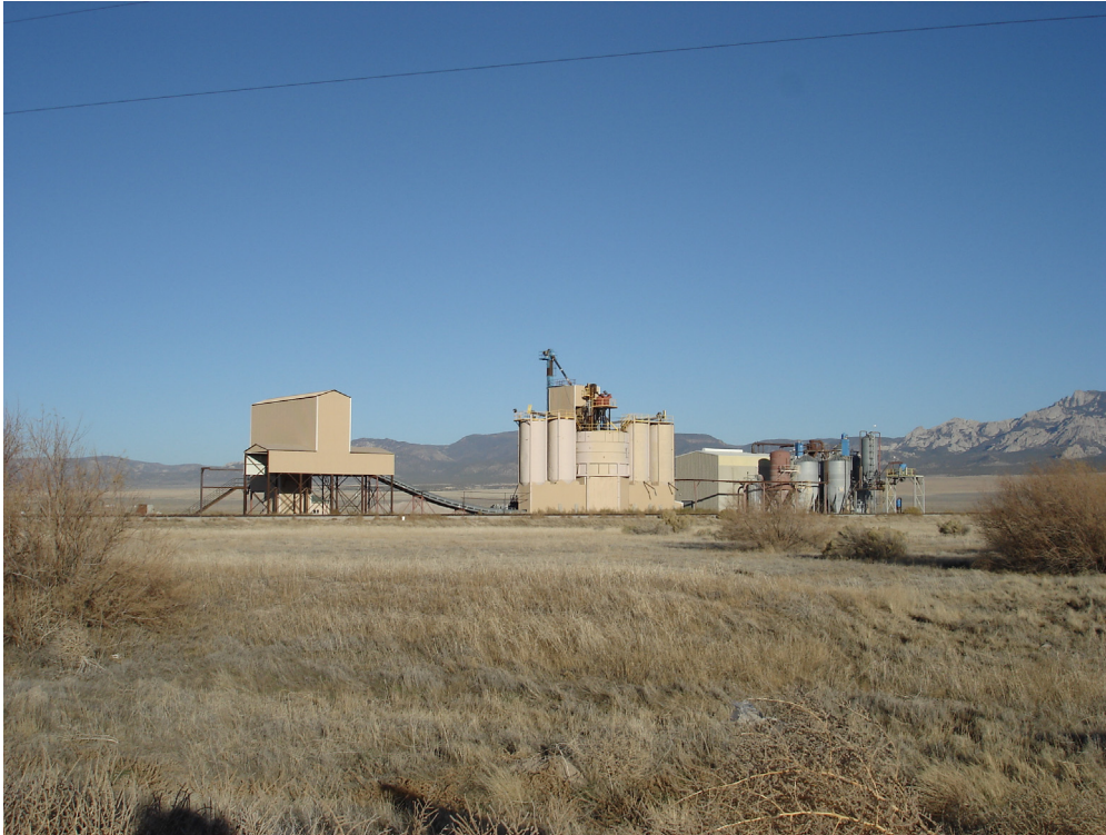
Figure 15. Imerys' Milford perlite plant, Beaver County, Utah.
