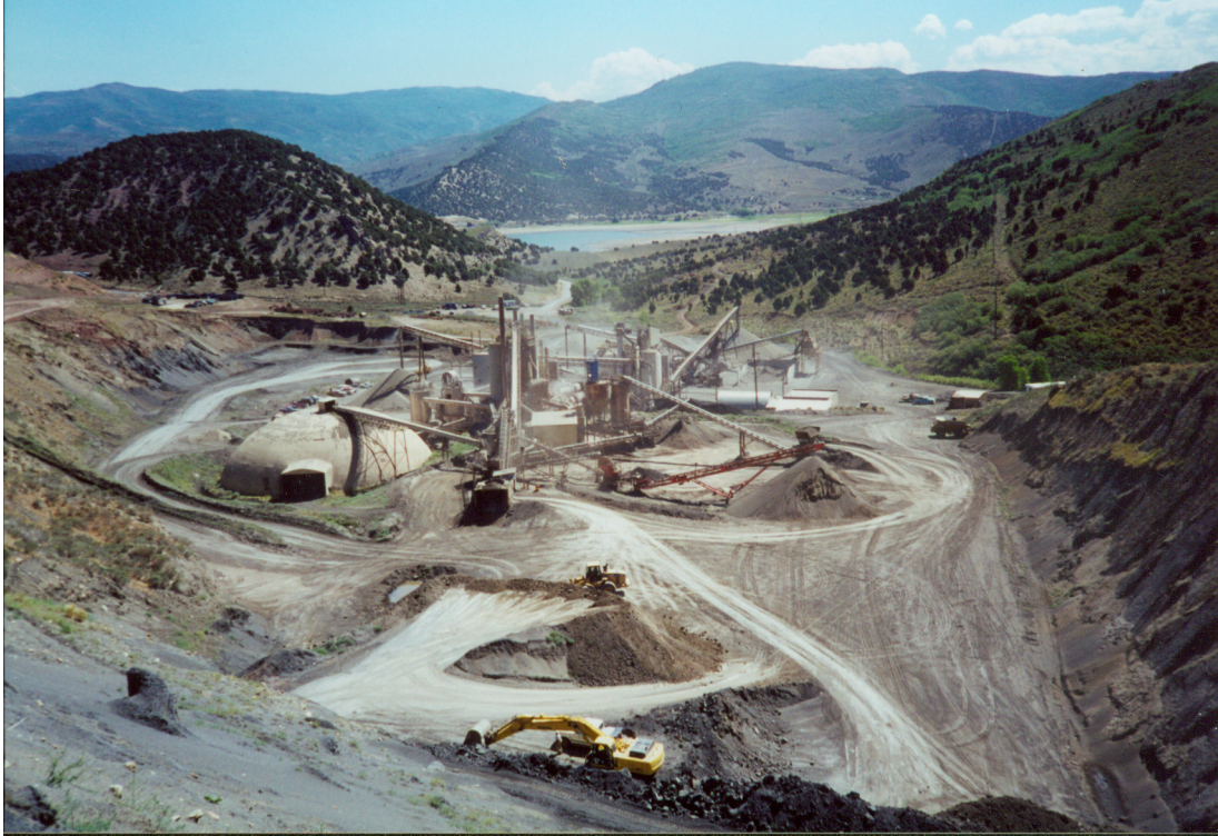
Figure 5. Utelite Corp.'s expanded shale plant in western Summit County; Rockport Reservoir is in the background (view is to the northeast).
