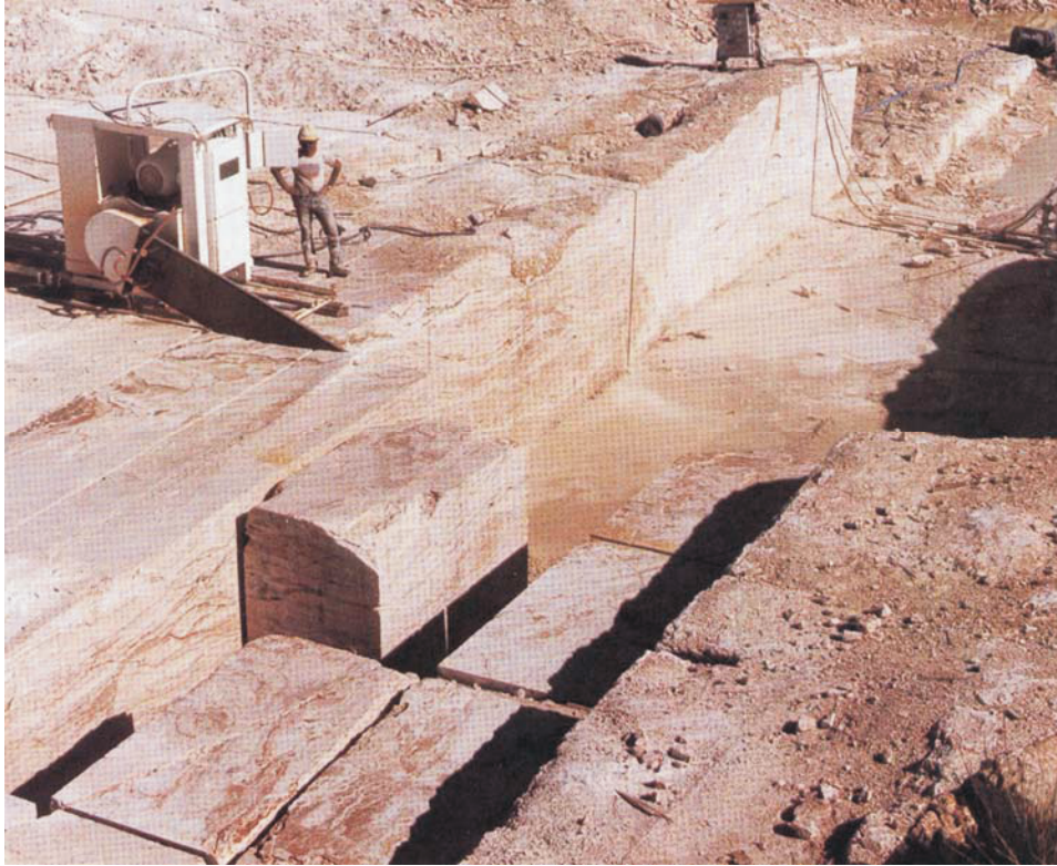
Figure 6. Scheherazade quarry at New Mexico Travertine quarries west of Belen, New Mexico. Diamond-impregnated belt saw in operation cutting 1½-inch channel as deep as 10 ft. Wire saw is “pulling the floor” on block previously cut by belt saw. Photograph courtesy of Rocky Mountain Stone.
