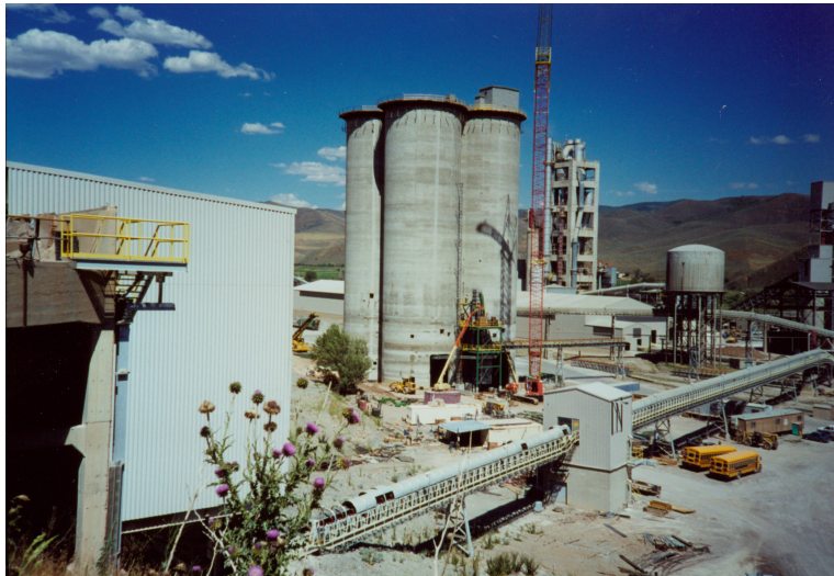
Figure 18. Holcim's Devil's Slide cement plant in Morgan County, Utah. The five-stage preheater/flash calciner tower is near the center of the photograph.
