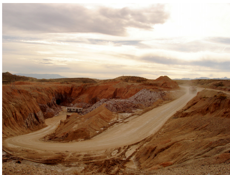
Figure 10. Portal of the South RCS underground rock salt mine in Sanpete County, Utah.
