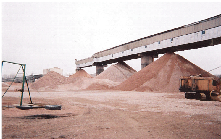
Figure 15. Upper photo: Train car and “big sack” quartzite loading area. Middle photo: Processing plant and quartzite storage area. Lower photo: Covered conveyor system depositing sized quartzite products.
