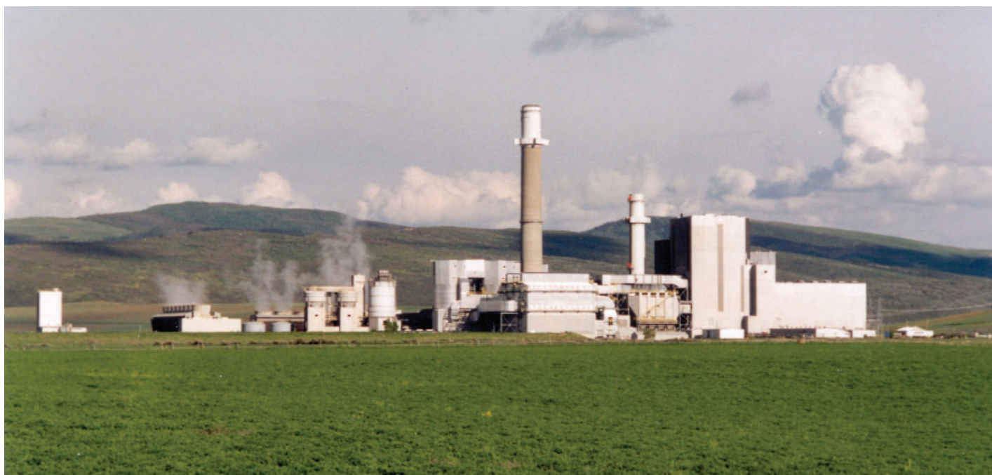
Figure 14. Xcel Energy Hayden Power Station.
