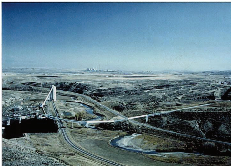
Figure 11. Empire Mine surface facilities with Craig Power Plant in the background. (Photograph courtesy of RAG American Coal Co.)
