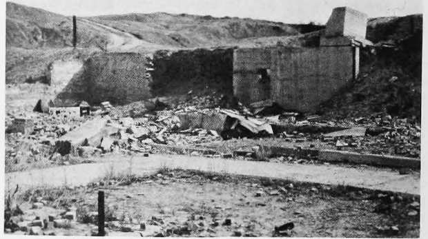
FIGURE 26b. Foundations of the dismantled Grand Junction Brick Company plant. Mancos Shale is exposed on the hills behind the old works.
