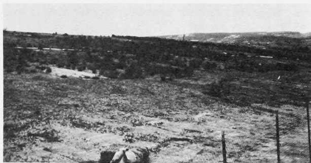
FIGURE 12. Uranium mill tailings near the Climax Uranium Company mill at Grand Junction. The 1.9-million-ton pile, although stabilized with a 6-in. grassed earth cover, is one of several Colorado sites that pose major disposal problems.
