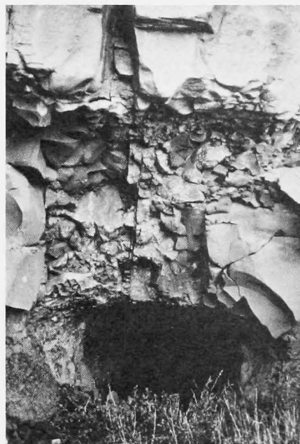
FIGURE 2. Lower (southeastern) adit of Copper Rivet Mine, Sinbad Valley. This tunnel leads to an upper tunnel and copper mineralization near the base of the massive faulted Wingate Sandstone.
