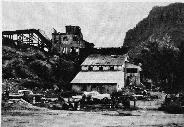
FIGURE 4. Abandoned vanadium mill of Gateway Alloys Company, Gateway. This plant processed Uravan belt vanadium ores between 1939 and 1945. In right background, massive Wingate Sandstone overlies Chinle and Moenkopi Formations.
