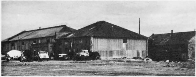
FIGURE 6. Main mill buildings of the Climax Uranium Company, Grand Junction. This complex in the country designed specifically to recover uranium, operated from 1951 to 1970.
