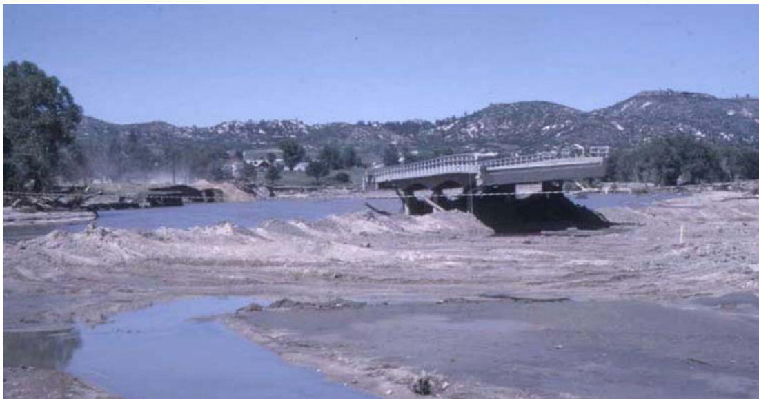
FIGURE 6. A bridge on Highway 67 south of Sedalia is washed out during the flood of 1965. Fragments of concrete, rebar, and other construction materials are still found in the alluvial deposits of Plum and West Plum Creeks. Cherokee Mountain is visible in the background. Photo by Charles Love; image courtesy of Douglas County Libraries.
