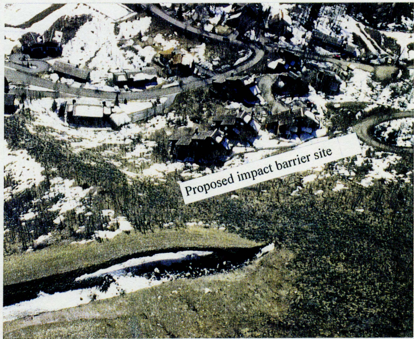
Photo #4. Location of proposed impact barrier or berm site. Note accumulation of rocks in existing ditch. The largest are 5 feet in diameter.
