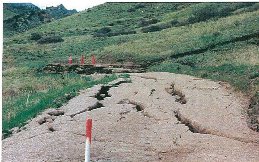
Photo 2. Bike path, damaged and offset by landslide, above Mesa Road. Note traffic cones in the background, on top of in-place path.
