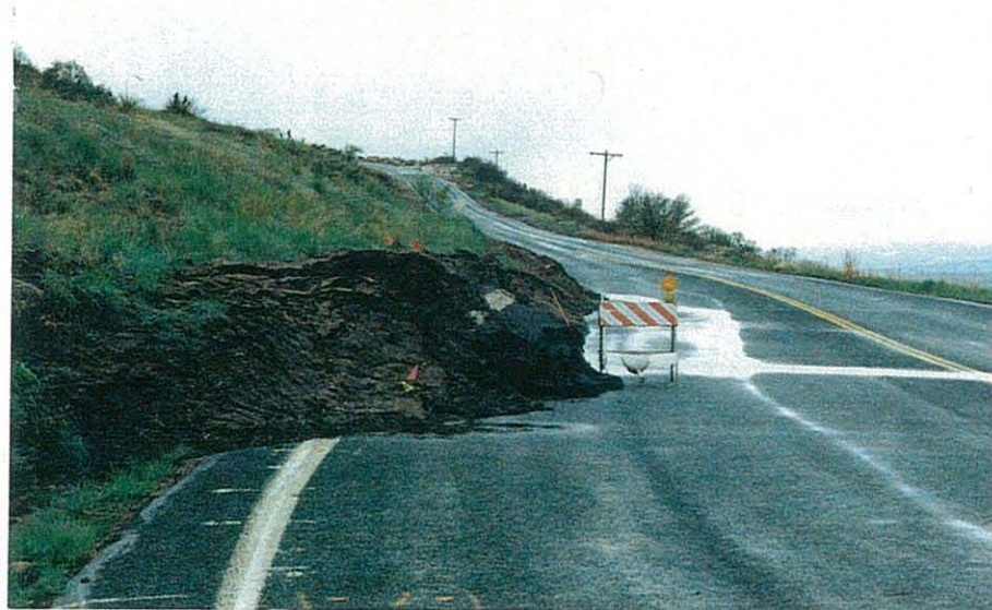
Photo 3. Toe of landslide encroaching on Mesa Road. Note white stripe on asphalt chunk in toe bulge left of barricade.
