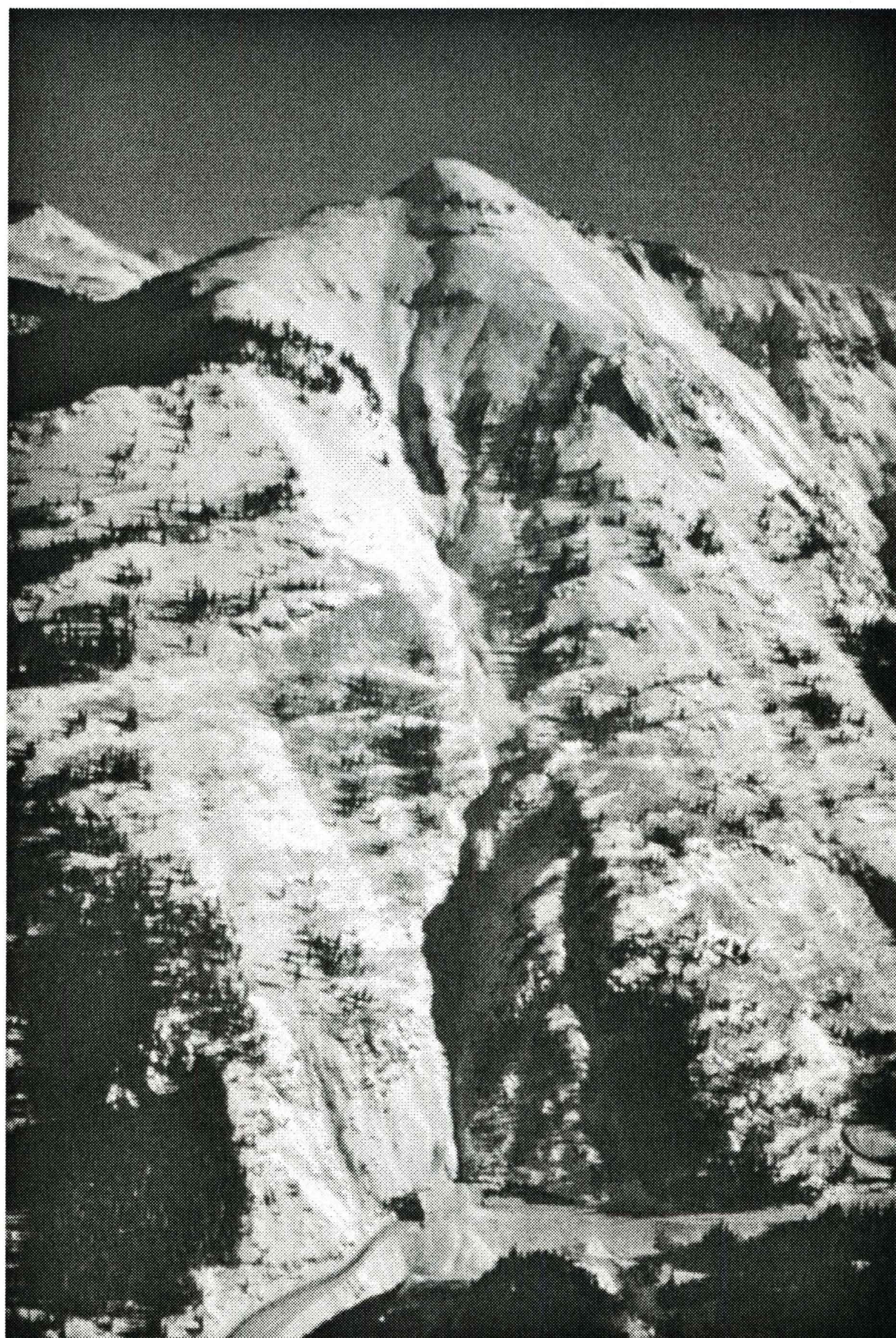
East Riverside Slide on the northwest side of Mount Abrams. Note snow-covered shed over State Highway 550 at bottom.
