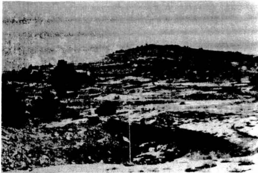
Figure 7. Collapse over room of Marshall No. 1 mine. The collapse area is approximately 15 feet by 30 feet and is about three feet deep. From five to ten feet of coal were extracted from this area at a depth of about 50 feet. Lower slopes of hill in background are also shown in Figures 6 (Area A), 8, 31, and 32. Locality 4, subsidence-inventory map.
