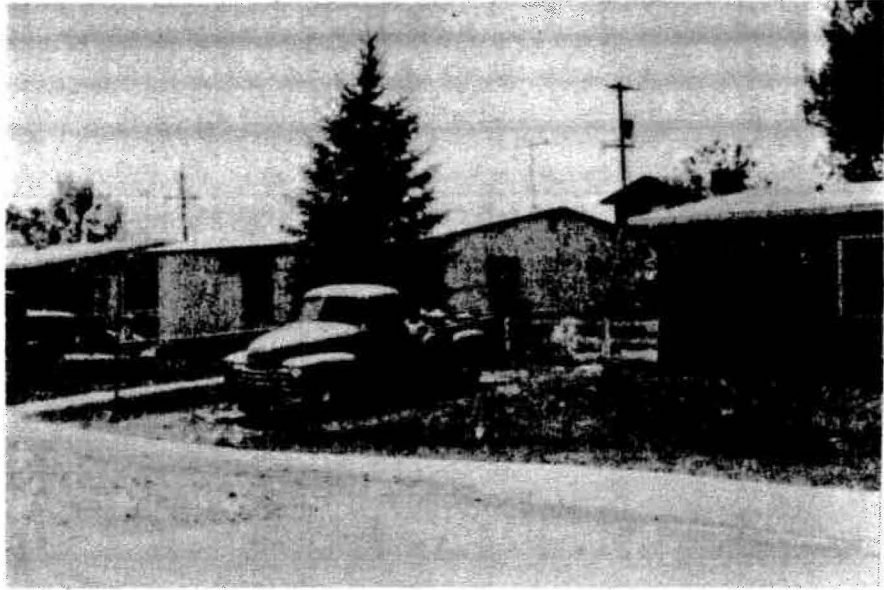
Figure 21. Subsidence over Strathmore mine, South Longmont Street, Lafayette. The most recent damage to the street has not yet been fully repaired. Note unpaved section of street and sagging sidewalk. The coal seam in this area of the Strathmore mine was quite thick, and the probable thickness of coal extracted was 20 to 25 feet. Depth of mining was 100 to 125 feet. Locality 55, subsidence-inventory map.
