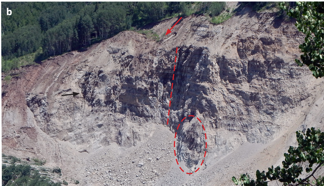
Figure 6(b). Photo of the east side scarp. Disturbed rockmass is the Green River Formation. Note sheared rock fabric and landslide displacement at side scarp shown by red arrow. Colluvial red soil is also seen in the scarp along left edge of photo. Red dashed line approximates major near-vertical shear zone. Dashed oval marks tightly spaced, near vertical shearing in rockmass.
