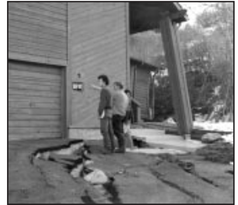
House condemned because of landslide damage
