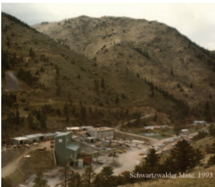
Figure 9. Schwartzwalder Mine, 1993. (Photograph courtesy of Jim Paschis)
