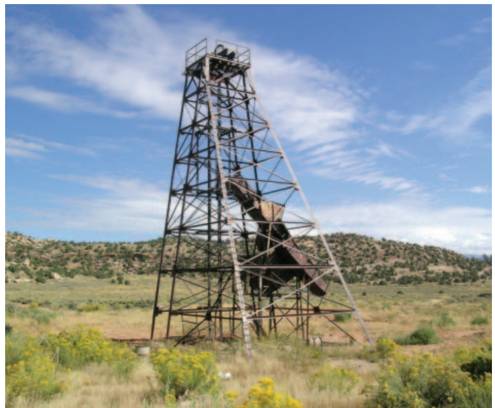
Figure 5. Long Park 16 Mine, near the site of the Radium Institute processing plant. (Photograph by Jim Cappa, 2005)
