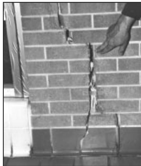
**Cracks in brickwork caused by swelling soils**
