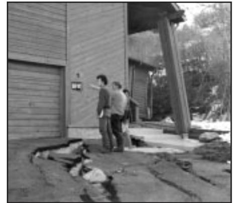
*House condemned because of landslide damage*
